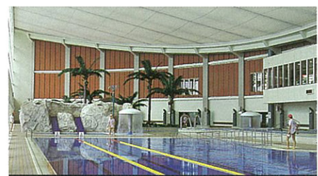
PLACE: Wall PURPOSES: Reduction of reverberation
