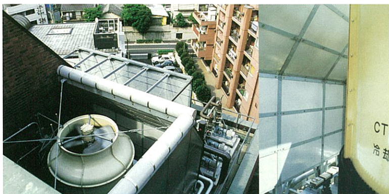
CT- 冷却 COOLING TOWERS PLACE: Noise barriers and noise reducers on the top of noise barrier PURPOSES: Decrease of noise level
